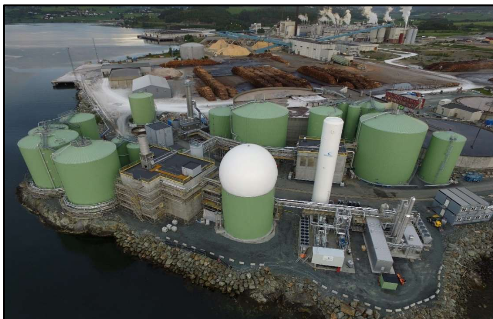
Picture showing Biokrafts plant in front and NSS papermill in behind.
