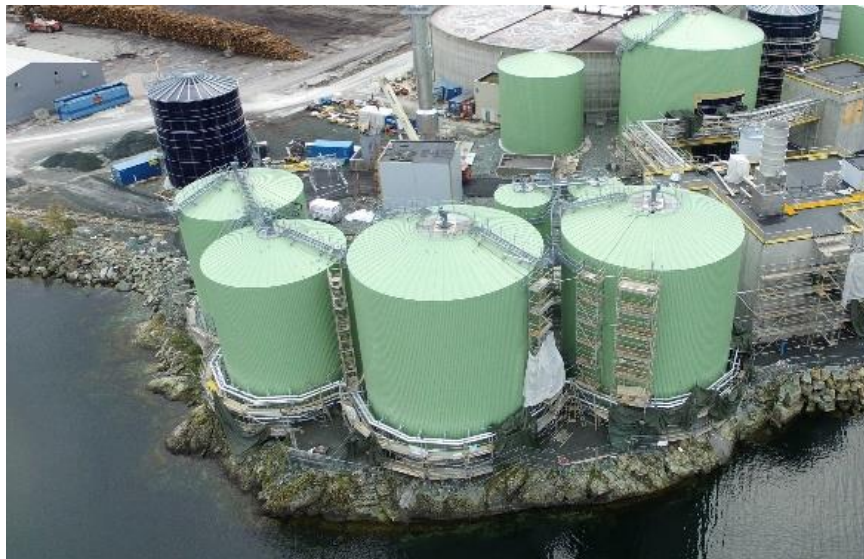
Figure 2 – Completed storage tanks
