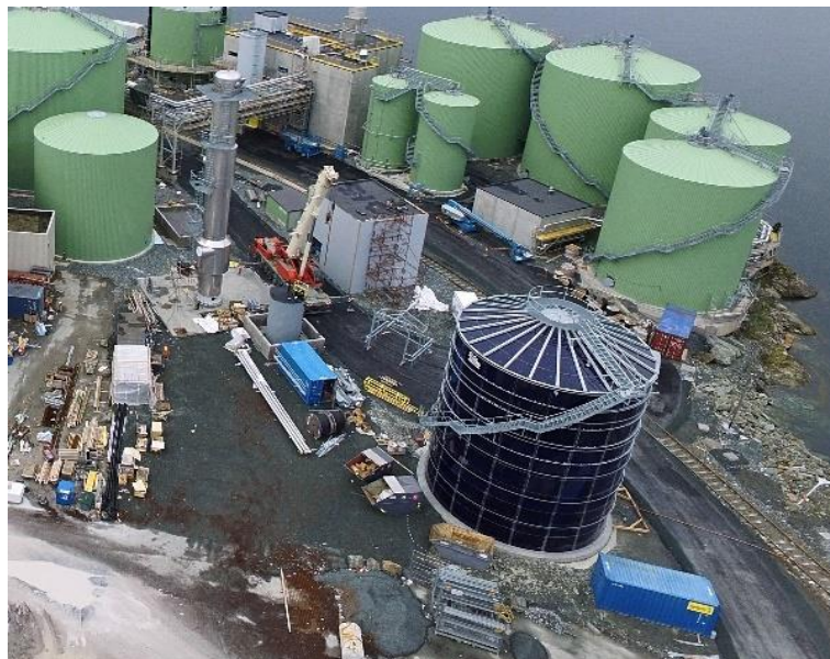
Figure 6 – Overview of area 4 under construction
